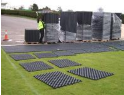
Sections arranged on the ground
