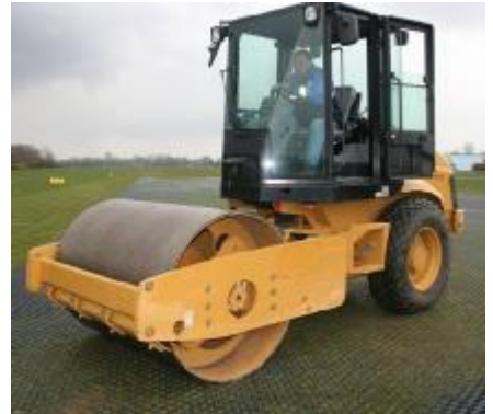
After several rows are laid out, they should be rolled, leaving the last row unrolled, ready for the next sections to be added
